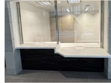
Accessible public information/service counter
