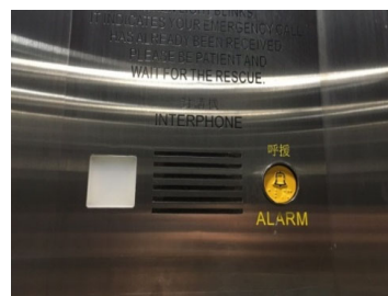
Emergency alarm push button in a tactile bell shape, Intercom and Audible indication to indicate the direction of travel and position of lift car
