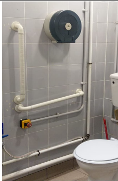
Horizontal and vertical grab rails adjacent to the water closet
