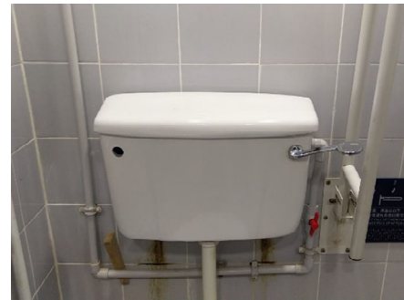
Flushing control mounted on the wide side of cubicle
