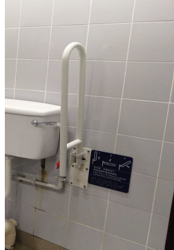
Folding grab rail on the wide side of cubicle adjacent to the water closet
