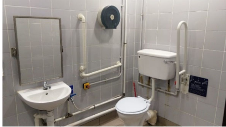
Horizontal and vertical grab rails adjacent to the water closet
