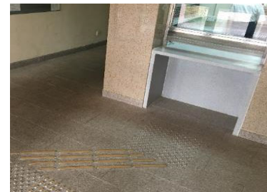
Accessible public information/service counter
