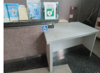
Accessible public information/service counter
